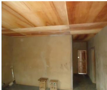
Interior of the building
